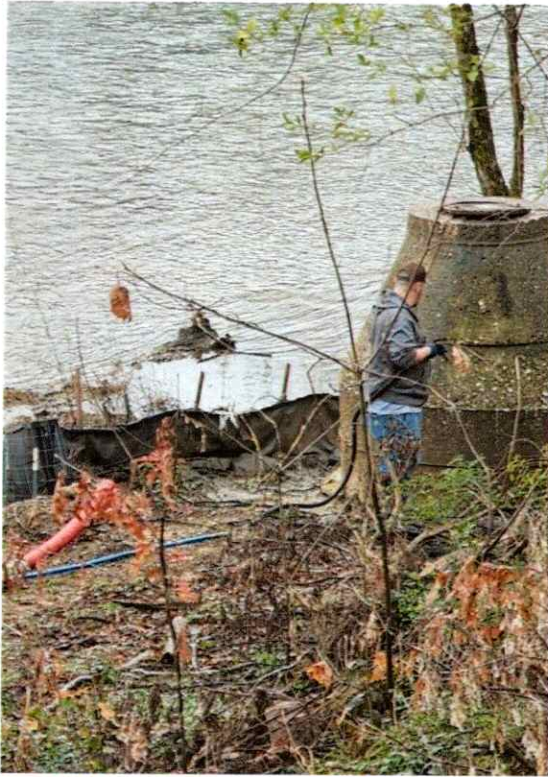
MH 1748 During Cleanup – 1/2/2025
