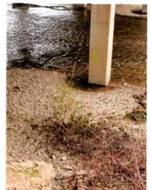
Sign Site 2 Removed 1/4/2025
